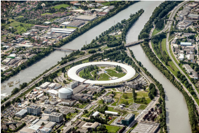
The European Synchrotron Radiation Facility (ESRF) in Grenoble. Image: © ESRF.
