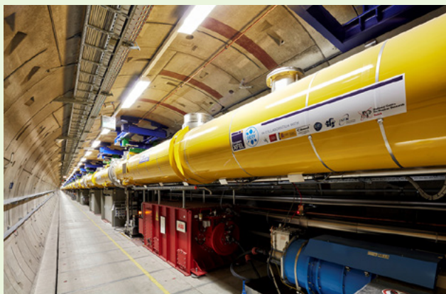
Inside the European XFEL tunnel. The yellow tubes are where electrons are accelerated.
