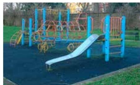
Figure 8: A playground surface composed of recycled rubber
