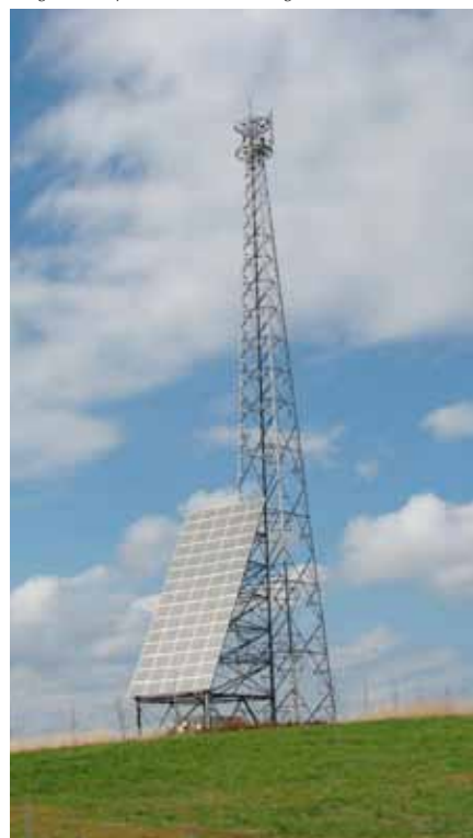
Mobile-phone base station powered by photovoltaics
